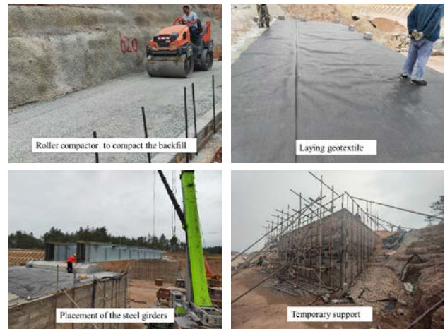
Fig. 27 Construction of the GRS-IBS
