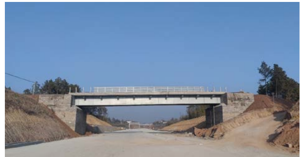
Fig. 28 Completed Tongyue overpass GRS-IBS
