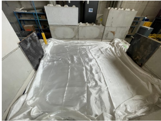
Fig. 2. Installation of the GTX.
