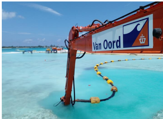
Fig 14. Pedestal excavator with floating pipeline
