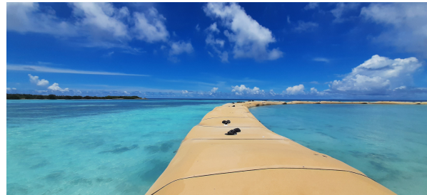
Fig 22. Non-woven geotextile to be placed against second layer geotube
