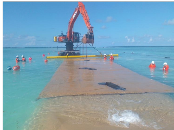
Fig 9. Pedestal excavator installing new geotube
