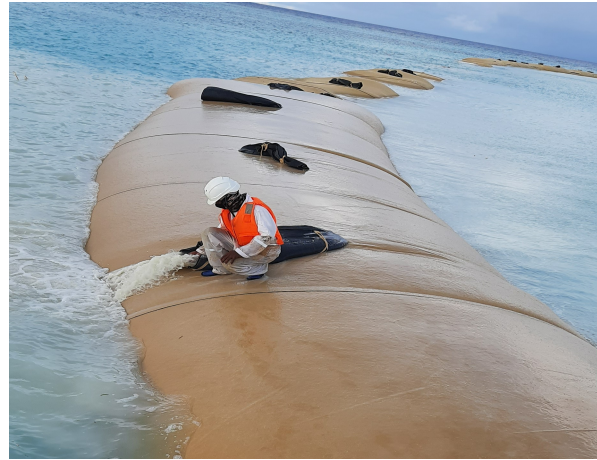
Fig 12. Supervision during installation
