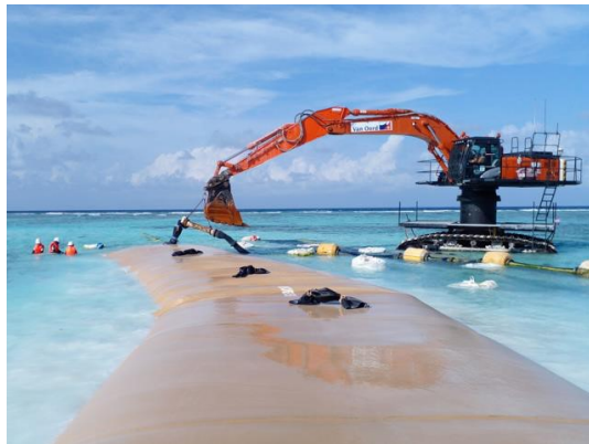
Fig 15. Pedestal excavator filling geotube
