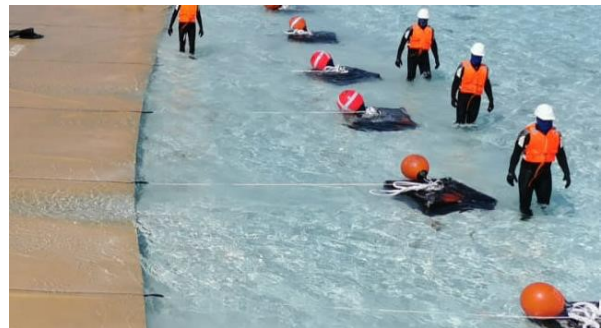
Fig 10. Workers assisting during installation
