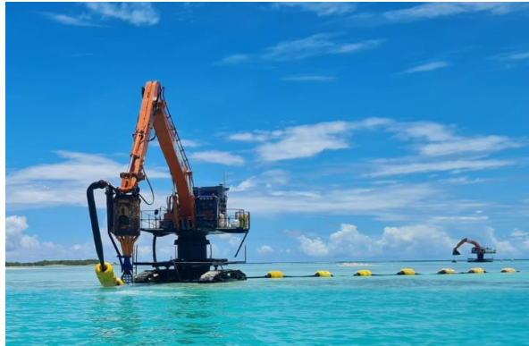
Fig 11. Pedestal excavator equipped with DOP and water jet pumps
