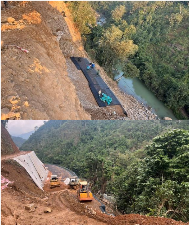
Fig.9. Images of the Mechanically Stabilized Earth project during construction
