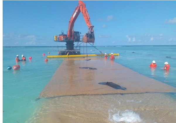
Fig 2 Tube Filling under progress
